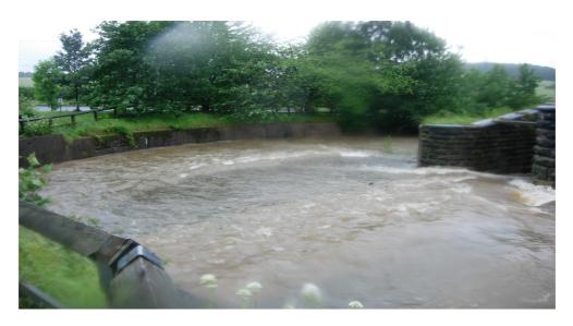
Figure 2 - Flow down 1943 spillway and original south spillway during the incident. Original south spillway is on extreme right of photograph.
