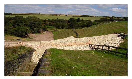
Figure 6 - Repaired scour hole after incident
