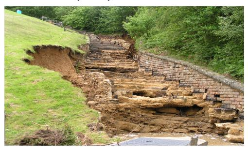
Figure 7 - Damaged spillway at Boltby in 2005
