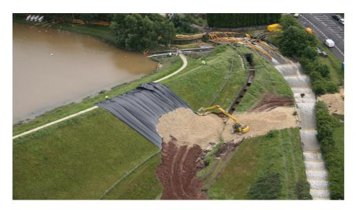
Figure 1 - Works in progress filling scour hole
