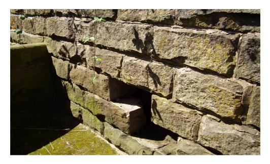
Figure 5 - Local hydrodynamic stone removal. Note also general condition of wall.
